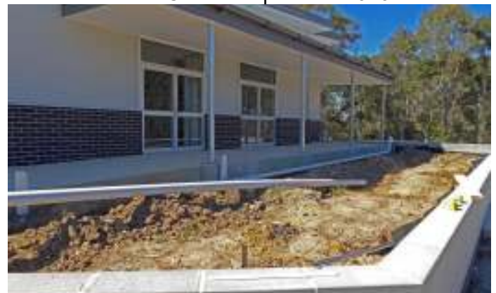
Western side of Church September 2016
